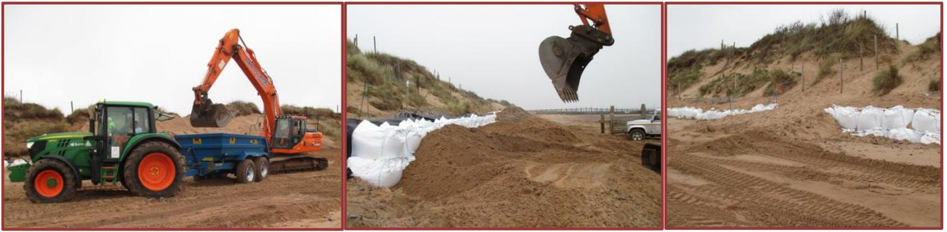
In order to minimise erosion of the dunes before the beach recharge in the summer, temporary protection measures have been put in place. Temporary sand filled bags have been placed in front of the dunes. These bags will be removed before the beach recharge. Wherever safe to do so, beach access points have been reinstated.
