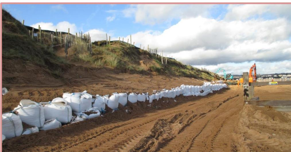
Some of the stone excavated from the gabion baskets is being used to create temporary platforms on site to allow other elements of work to proceed. Ultimately, all gabion stone will be removed from the beach and taken off site for re-use.
