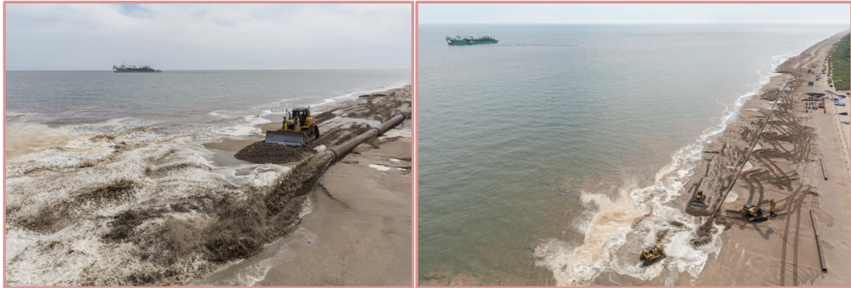
Beach replenishment on the east coast of the UK, using similar methods to what will be used at Dawlish Warren
