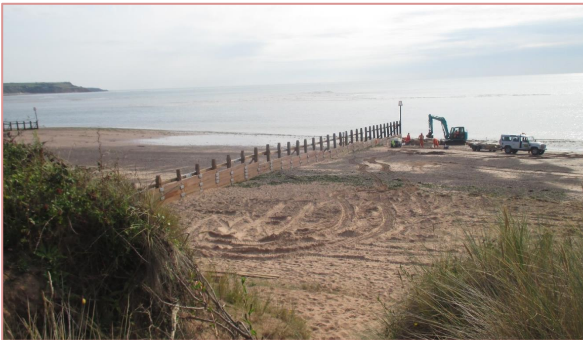
Completing refurbishment of Groyne 9
